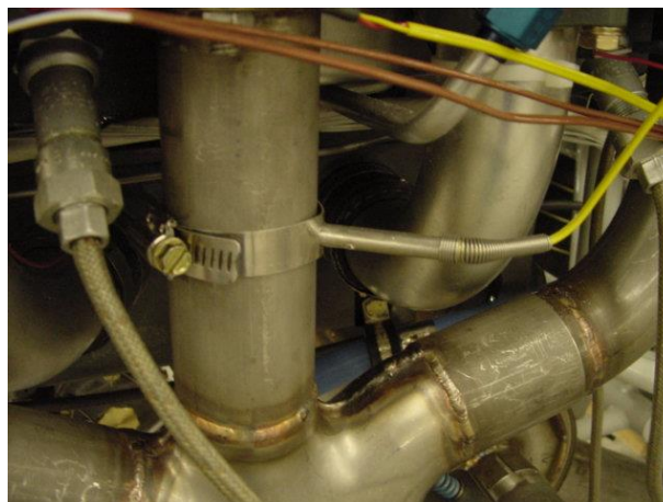
EGT Probe Location
